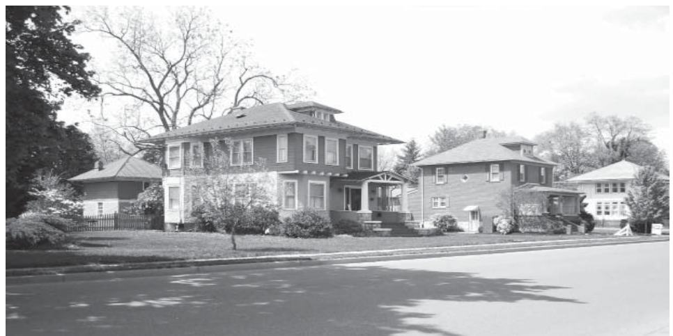
West Martinsburg Historic District, Berkeley County
