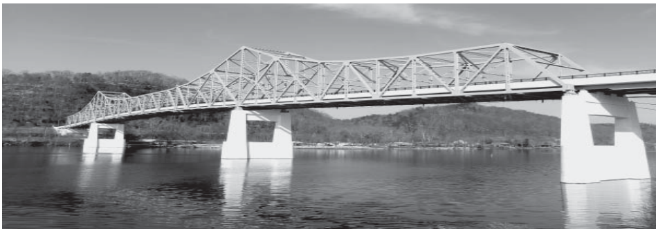
Winfield Toll Bridge, Putnam County
