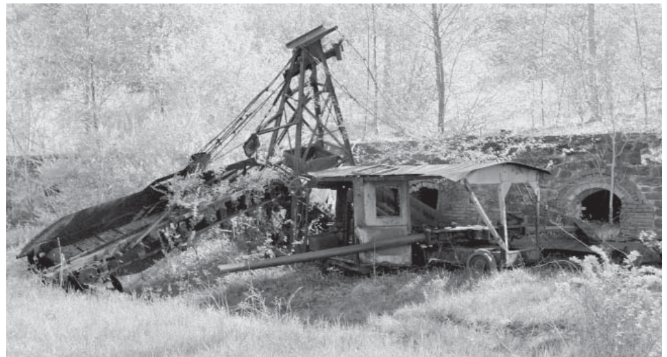
Coke Oven and Equipment - Bretz, Tucker County
