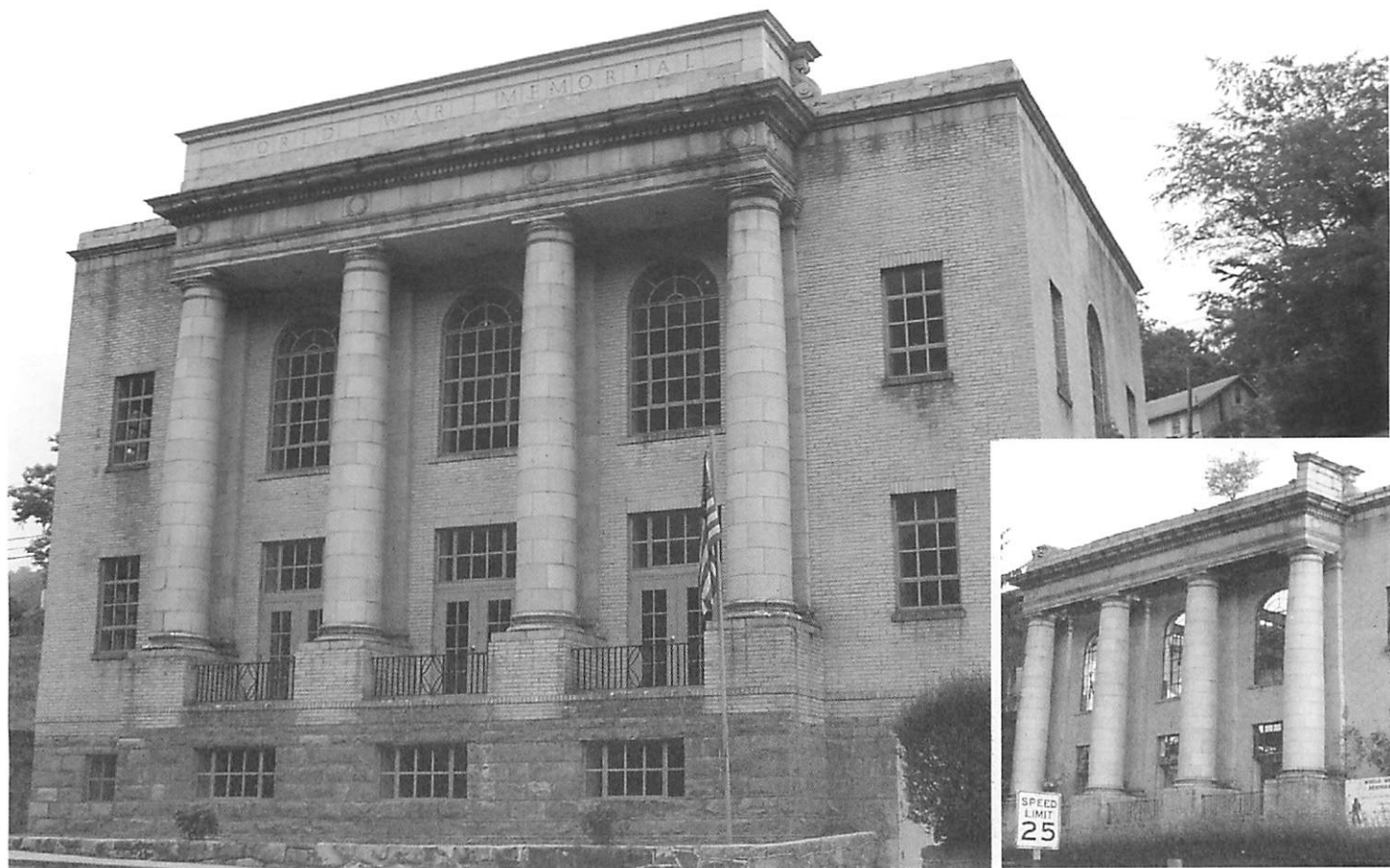
The restored Kimball War Memorial. Inset: Before renovations.
